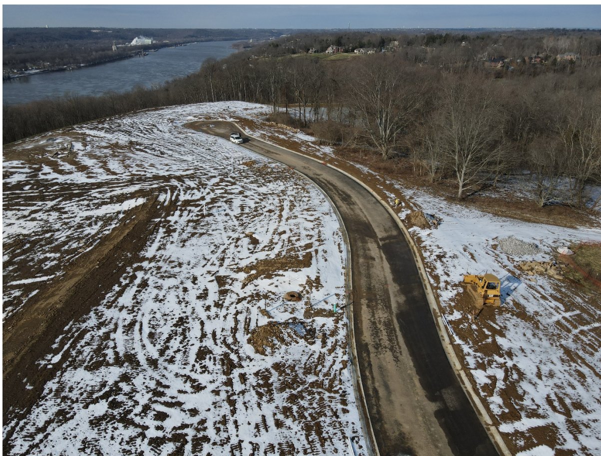
View of site from above (Courtesy of Anderson Township)
