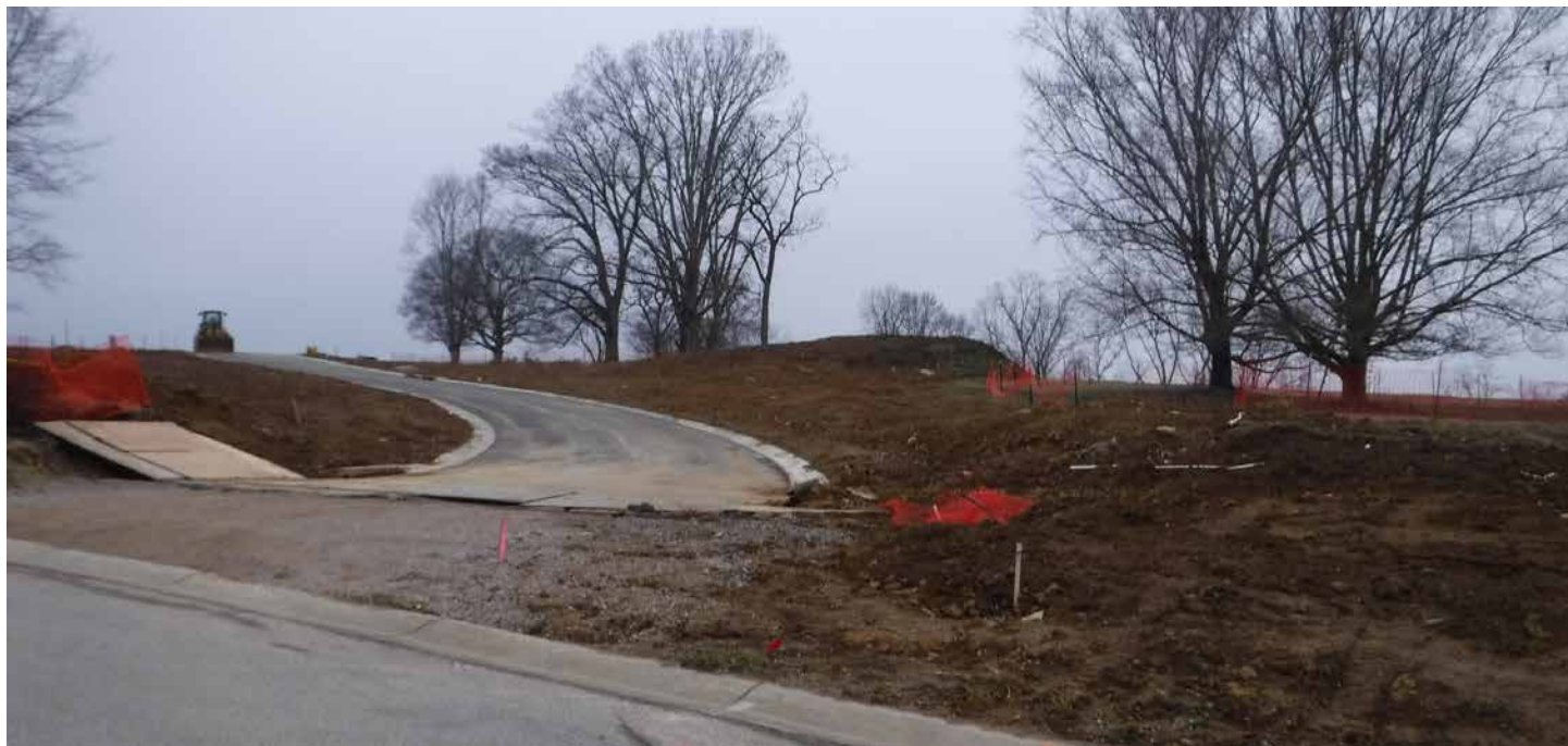
View (south) of from Ayers Road (Courtesy of Anderson Township)
